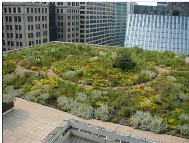
Figure 12.1 - Extensive Green Roof
