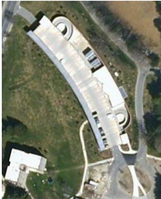
Figure 9.1 - Satellite image of parking deck during construction
